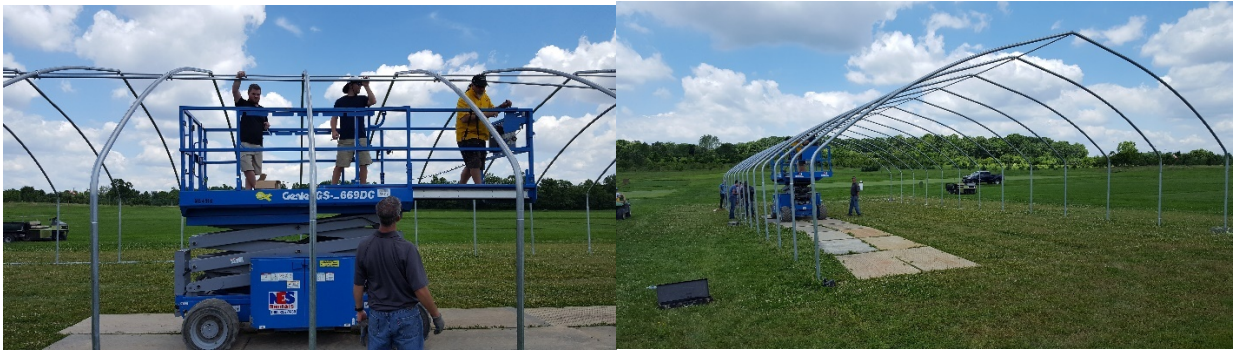
SHELTER CONSTRUCTION AT THE UNIVERSITY OF MARYLAND, COLLEGE PARK, MD
